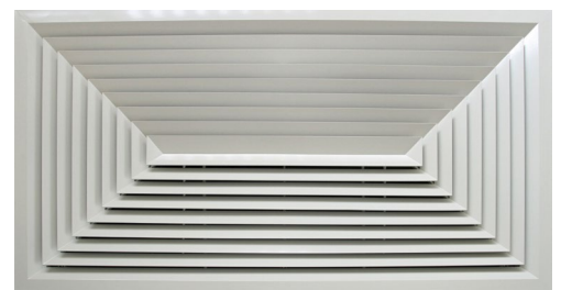
Flush Face Diffuser - Double Tile 4 Way Blow
